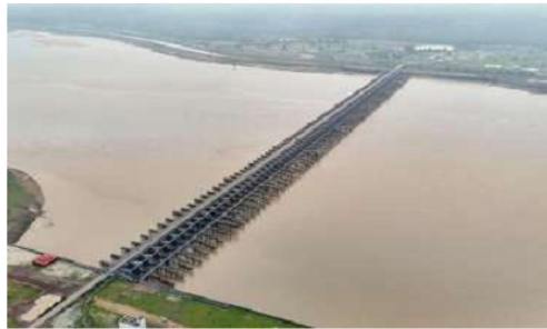
One of the barrages of the Kaleshwaram project on the Godavari.
